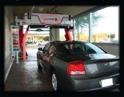
Arms flash RED, telling users to 'Stop for Washing,' and continue flashing until the end of the wash cycle
